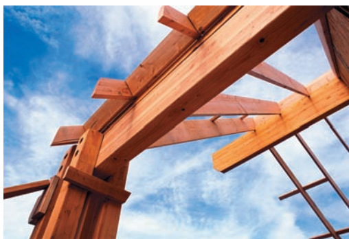
Photo 5.1 Timber beams used in residential dwelling.
