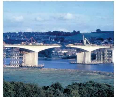
Photo 5.2 Nonprismatic cantilever beams of bridge during construction.
