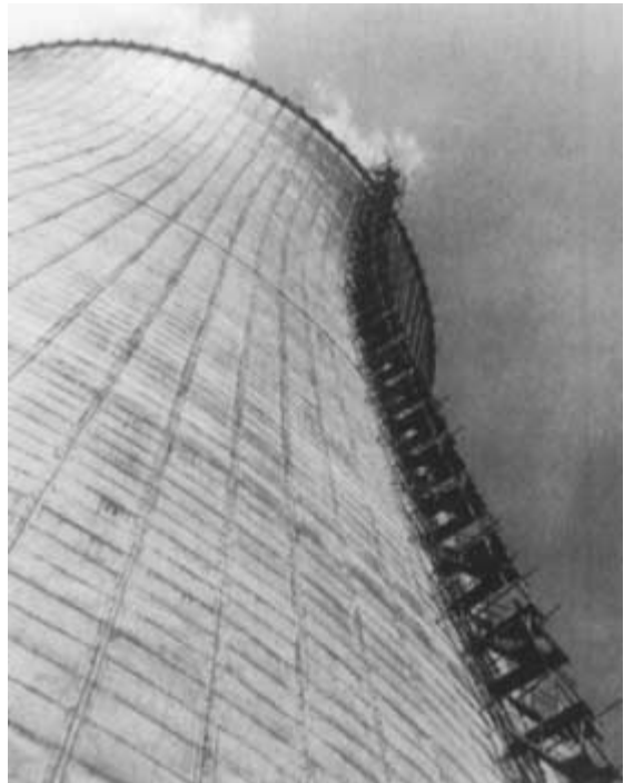
FIGURE 10.6 “Tubelox” tube and coupler scaffolding with integral step units for access to 330-ft-high curved stack. The step units are available with guardrail and midrail panels, plus the opportunity of positioning landing or rest platforms at any desired level.
