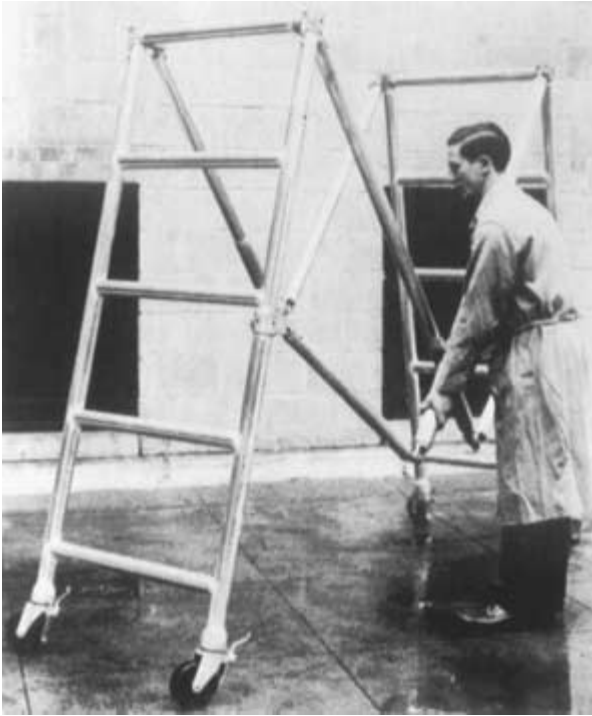
FIGURE 10.3 Folding aluminum ladder scaffolds are designed so that the end frames will not fall over at any point during the erection or dismantling process. It is a completely free-standing unit at all times.
