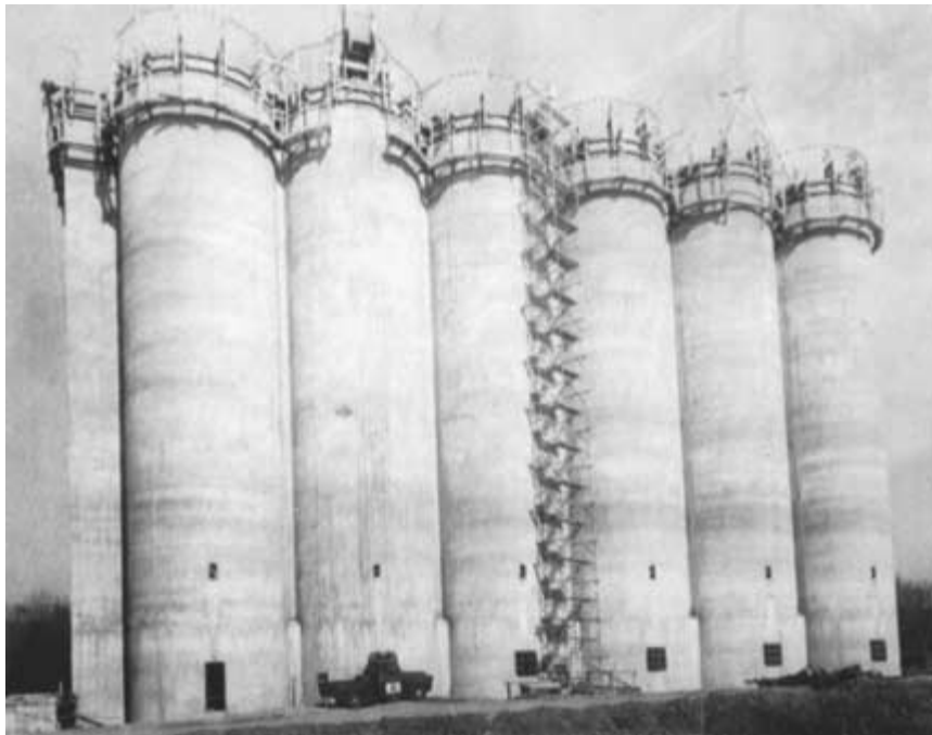
FIGURE 10.7 Trouble-saver sectional scaffolding with built-in step units for silo access during construction. Similar installations are quickly erected for many industrial maintenance operations when the safe, speedy vertical movement of persons is needed. ( The Patent Scaffolding Co., Inc. Photo by Tracy O'Neal. )
