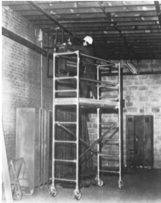
FIGURE 10.10 Aluminum ladder scaffold. Basic unit consists of 6-ft ladder frames, diagonal braces, platform, and adjustable casters. Note use of guardrails, midrails, and toeboards.
