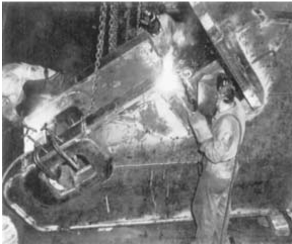
FIGURE 1.2 Long delivery time prompted welding of this cast iron punch-press frame.
