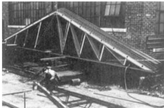
FIGURE 1.5 Maintenance department fabricating trusses for plant expansion. Trusses made from channels and angles. A jig was laid out on plate in the plant yard.
