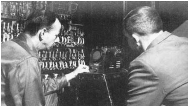
FIGURE 5.2 Cathode-ray-tube oscilloscope typifies the more advanced instruments that maintenance technicians use in analyzing the performance of modern elevator equipment. Checking the operation of automated elevators with great accuracy, the technician can promptly make any necessary adjustments to restore “like-new” service.
