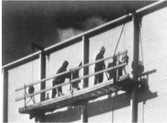
FIGURE 10.8 Safety swinging scaffold (two-point suspension). Utilizes steel-wire rope with ratchet-action raising and crack-handle lowering. Note use of guardrails, midrails, and toeboards. Similar scaffolds are also available with power machines and aluminum platforms. Safety belts, lifelines, and lanyards must always be available and used on all swinging scaffolds.
